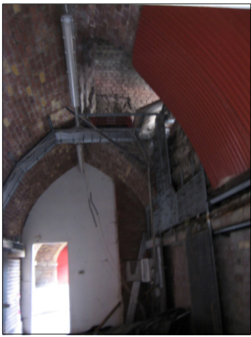
EXISTING HOARDINGS, FITTINGS & SERVICES - Redundant from previous uses and to be stripped out.
